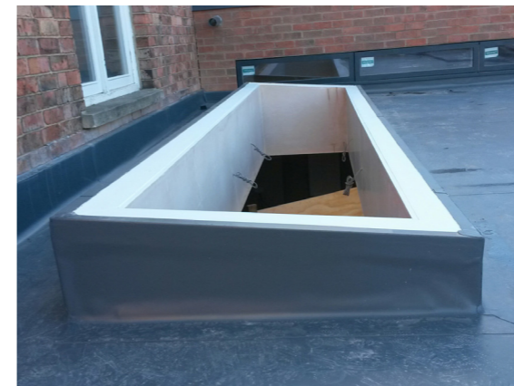
Upstand complete with weathering
