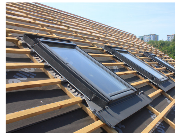
Roof window install prior to flashing and tiling
