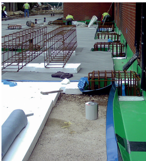
Fosroc 'Engage' installed under slab
