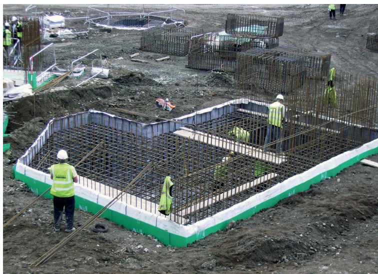
Hydromat sheet connected inside corriform formwork to proof high water table
