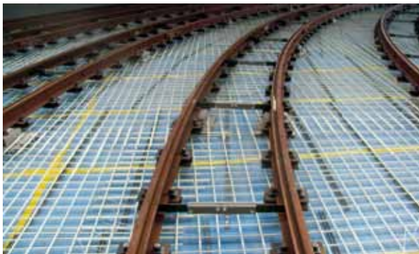
Floor slab railway depot Basel, Switzerland
