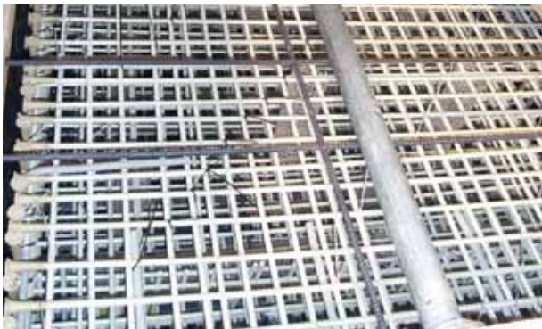
Foundation block at the IBM Nanotech-Center in Zurich, Switzerland
