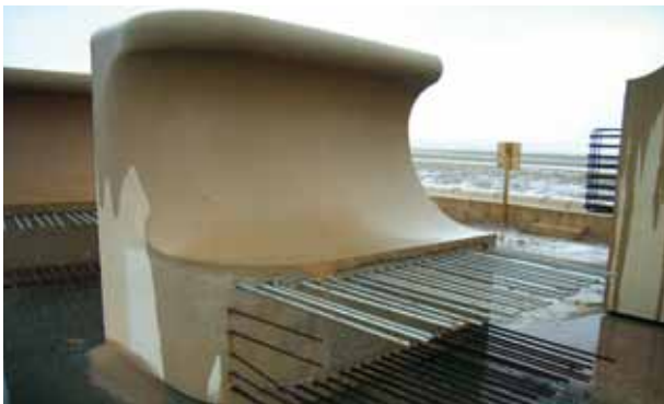
Precast concrete elements for coastal defense project Blackpool, UK
