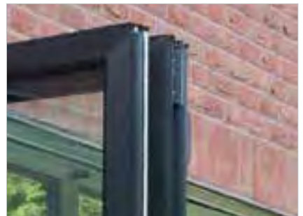
Magnetic door stops for a neat fold
