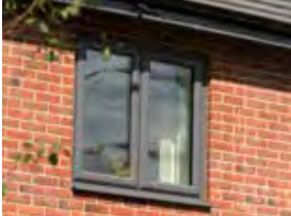
Chamfered casement windows
