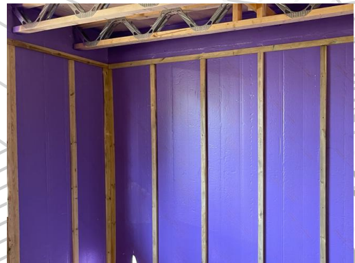
5.2.2 Service battens installed over Passive Purple Internal
