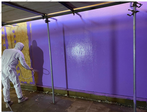
5.2.1 Spraying on to OSB board
