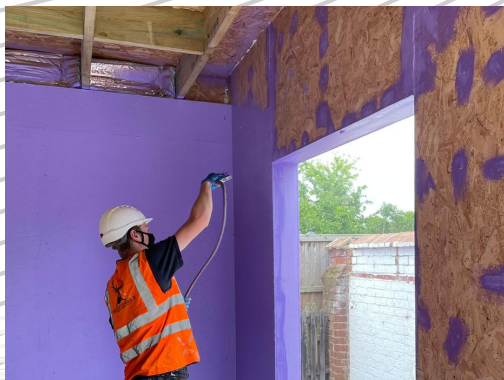
5.2.3 Prepped walls by brushing joints between boards and nail heads
