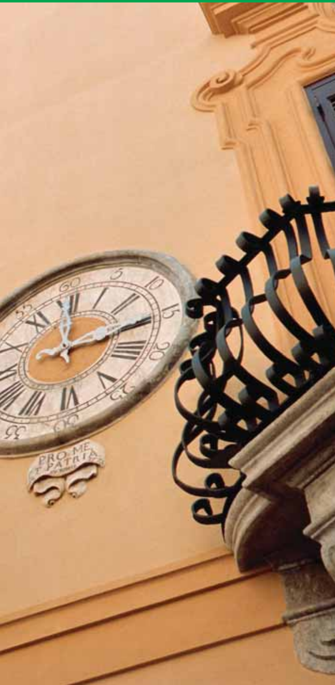
Ferro Palace - Trapani - Italy Reparation and decoration of the façade with: MAPE-ANTIQUE MC, MAPE-ANTIQUE RINZAFFO, SILEXCOLOR PRIMER, SILEXCOLOR TONACHINO
