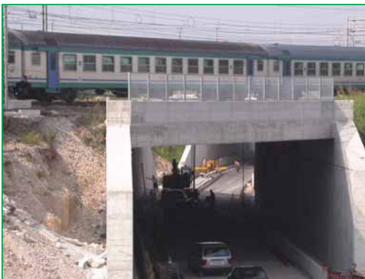
Fenilone railway underpass - Verona - Italy Structural reparation and consolidation with: ADESILEX PG1, CARBOPLATE, MAPEWRAP 11, MAPEWRAP 12, MAPEWRAP C UNI-AX
