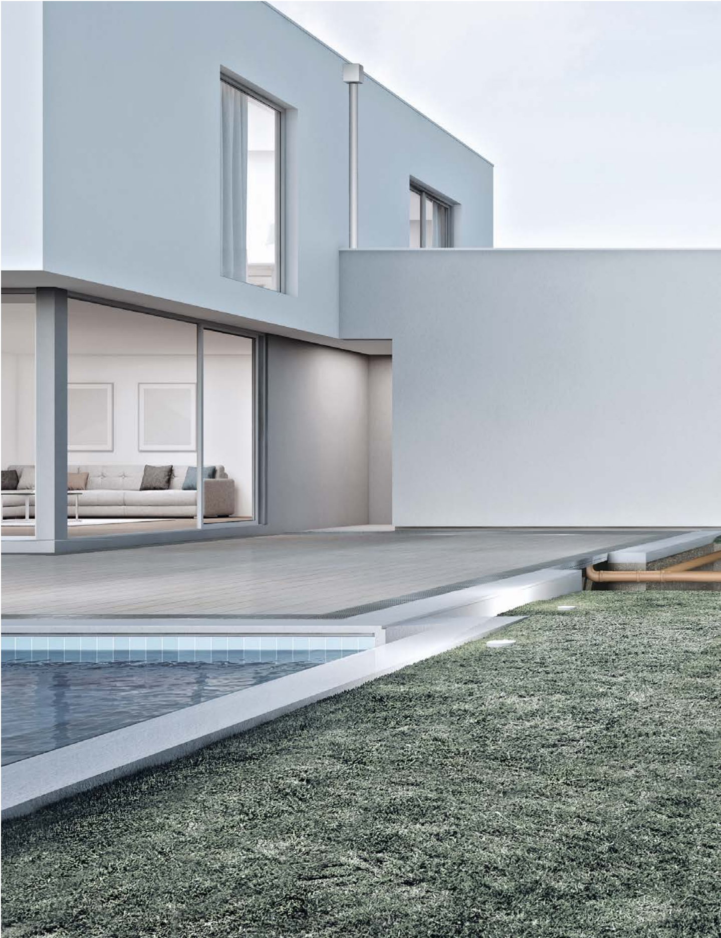
Seepage of rainwater from the terrace and roof
