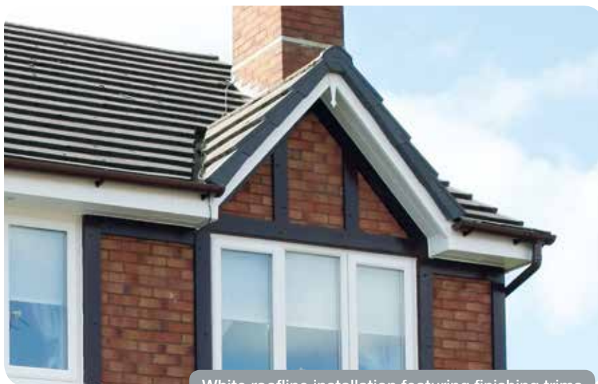
White roofline installation featuring finishing trims
