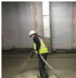
NB1 SPRAY APPLICATION
