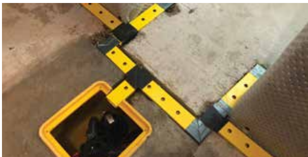
BASEMENT DRAINAGE TO COMPLIMENT TYPE C SYSTEM
