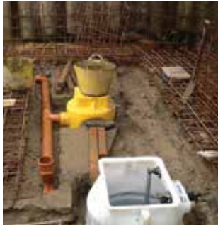
RESIDENTIAL BASEMENT DRAINAGE
