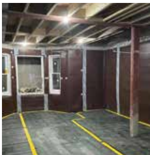
TYPE C WATERPROOFING & GROUND GAS PROTECTION
