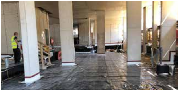
GROUND GAS PROTECTION AT COMMERCIAL STRUCTURE
