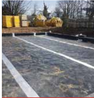
PRO TITAN INSTALLATION
