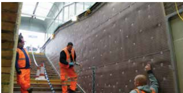
DAMP PROOFING - LONDON UNDERGROUND STATION
