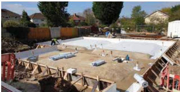
DELTA DUALPROOF INSTALLATION
