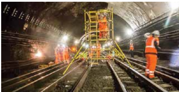
RESIN INJECTION - LONDON UNDERGROUND
