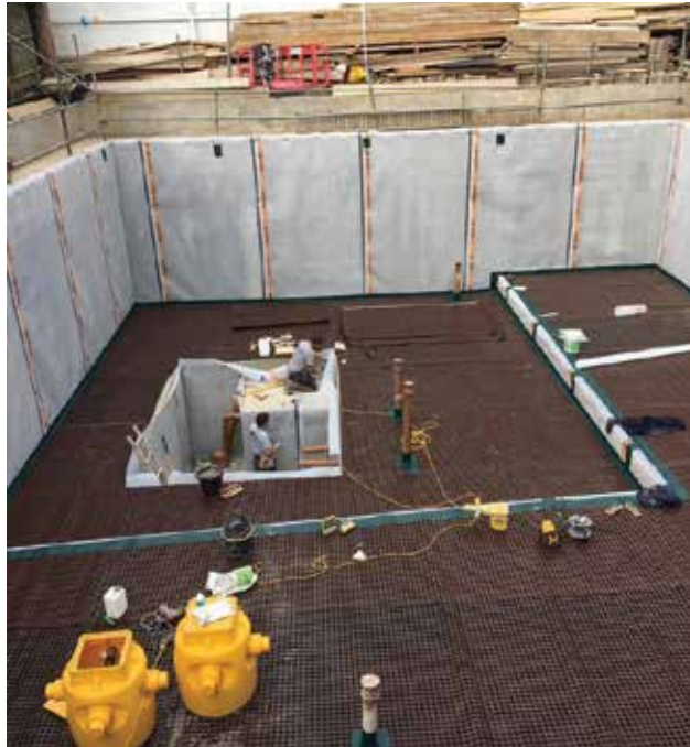
DELTA DUAL V6 INSTALLATION ON SITE
