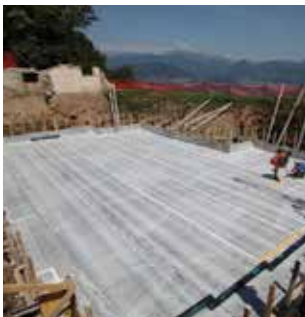
DELTA AMPHIBIA INSTALLATION
