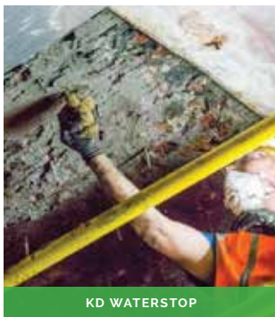
RESIN INJECTION - LONDON UNDERGROUND
