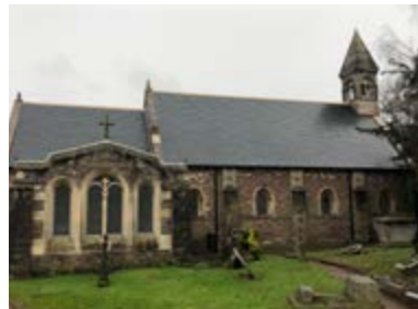
The Parish Church of Saint Mary's Malpas 4 Llanover Cl, Newport NP20 6GR
