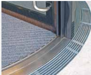
From left to right: – Laser sensor for precise recognition of persons or objects. – Safety sensors automatically adjust the door speed to the flow of persons. – Outside entrance detail with circular drainage steel grid. – Antislip and dirt absorbing floor mat.
