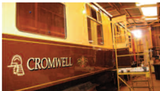
Heritage railway carriage refurbishment (Rampart Engineering Ltd)
